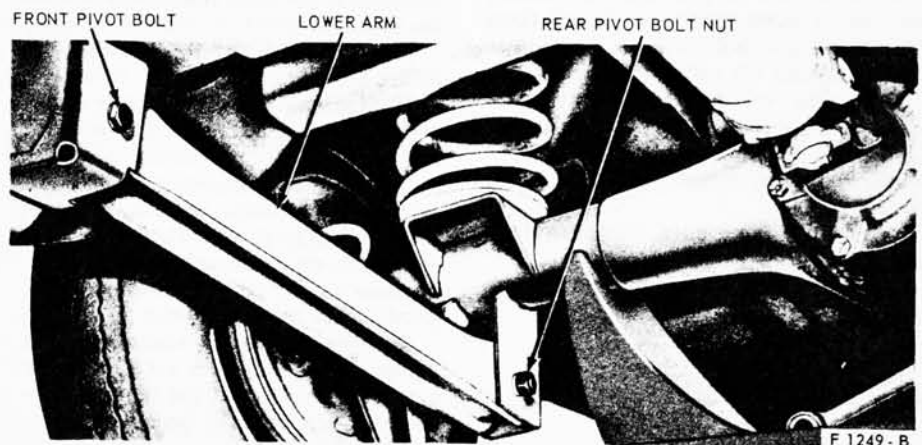
FIG. 6—Rear Suspension Lower Arm Installed
